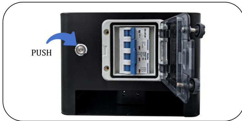
Figure 32 The Power Switch Of Battery Systems
